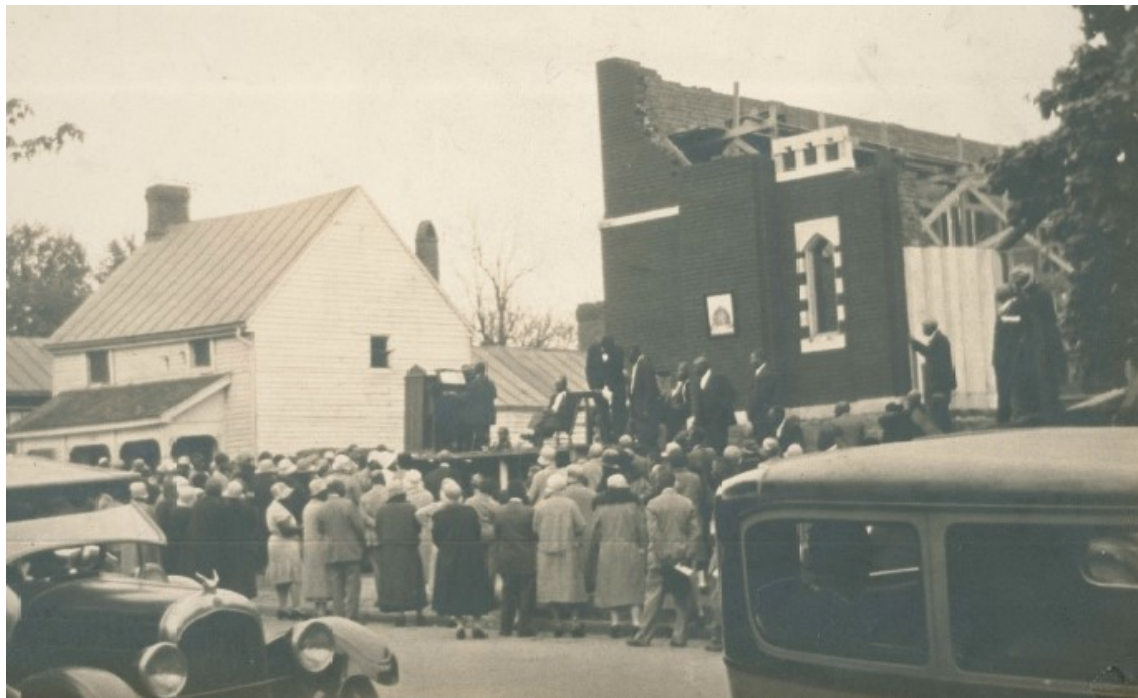
First Baptist Church during construction.
